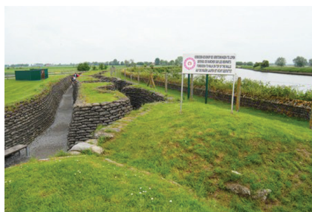
Fig. 1 - The Trenches of Death (Boyou de la Mort, Dodengang), near Dixmude (Belgium). The level of the water table impeded digging, and trenches were raised by piling sandbags.
